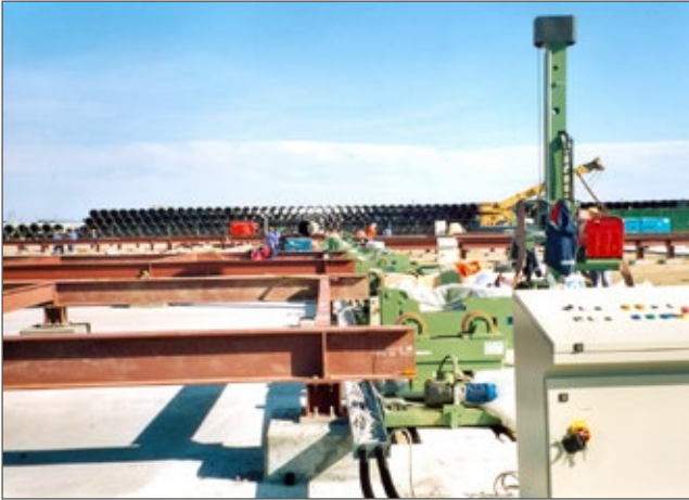
BTC (Baku>Tiblisi>Cheyang) pipeline: DJ yard at Yevlah Camp - Azerbaijan
